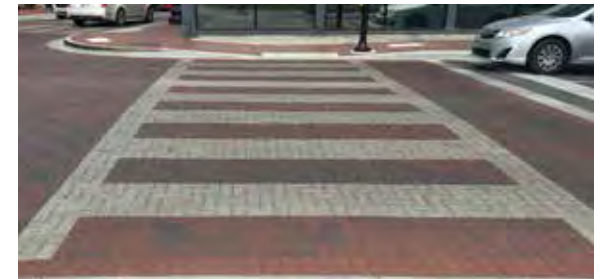
Crosswalks at the intersection of Main Street & Madison show how color and textures can help crosswalks stand out.
