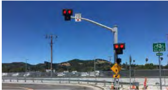
HAWK Signals allow pedestrians to stop traffic to cross streets. Source: City of San Rafael
