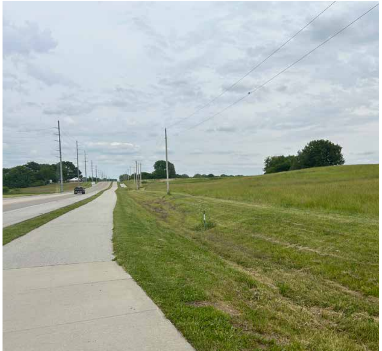
A multi-use trail runs along the southern side of Worthsville Road from the I-65 interchange to Griffith Road.
