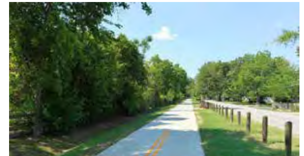
Shared-use paths can be separated based on traffic flow or user type.
