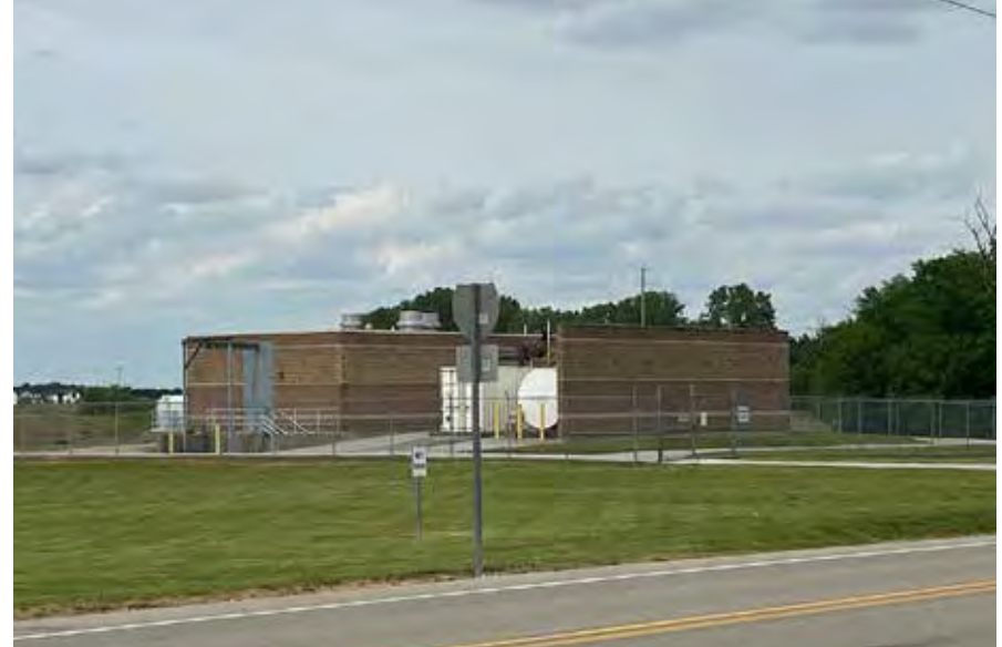
The Hurricane Creek lift station on the north side of Worthsville Road is in place to serve anticipated growth in the area.
