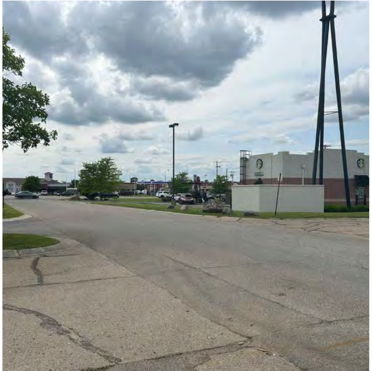
The block at the corner of Emerson Avenue and E Main Street holds major infill potential and internal connectivity improvement after the demolition of the Red Carpet Inn.
