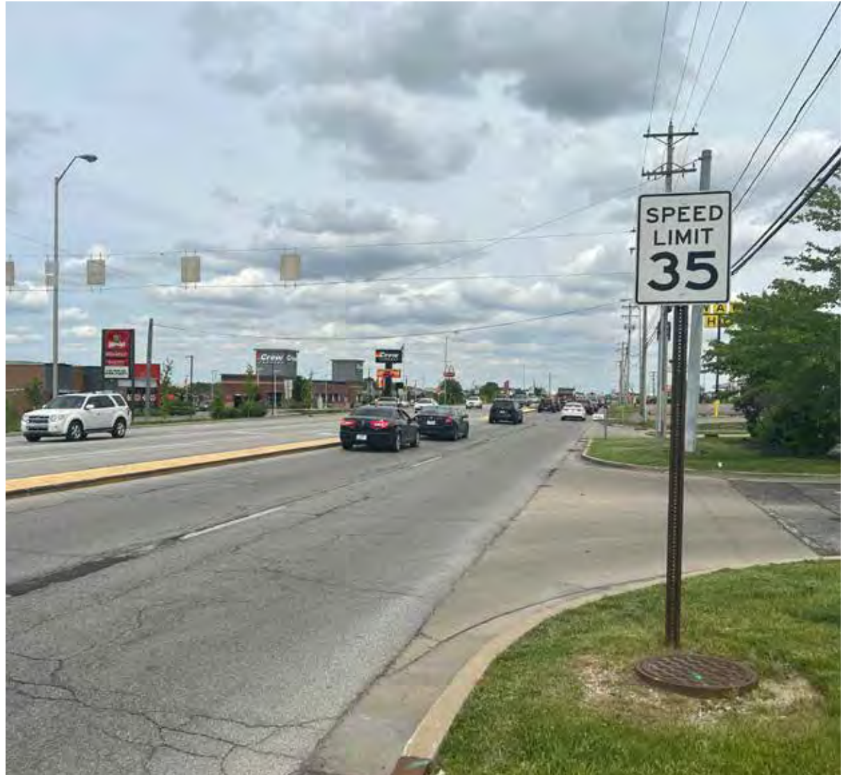
An E Main Street & I-65 interchange study was started in 2024 in repose to major traffic congestion on Main Street during high-traffic times, backing up to Emerson Avenue in some cases.
