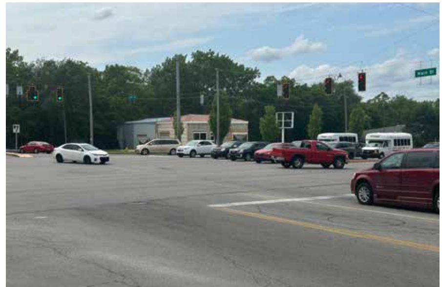
The intersection of Main Street and U.S. 31 experiences back-ups during peak travel times.
