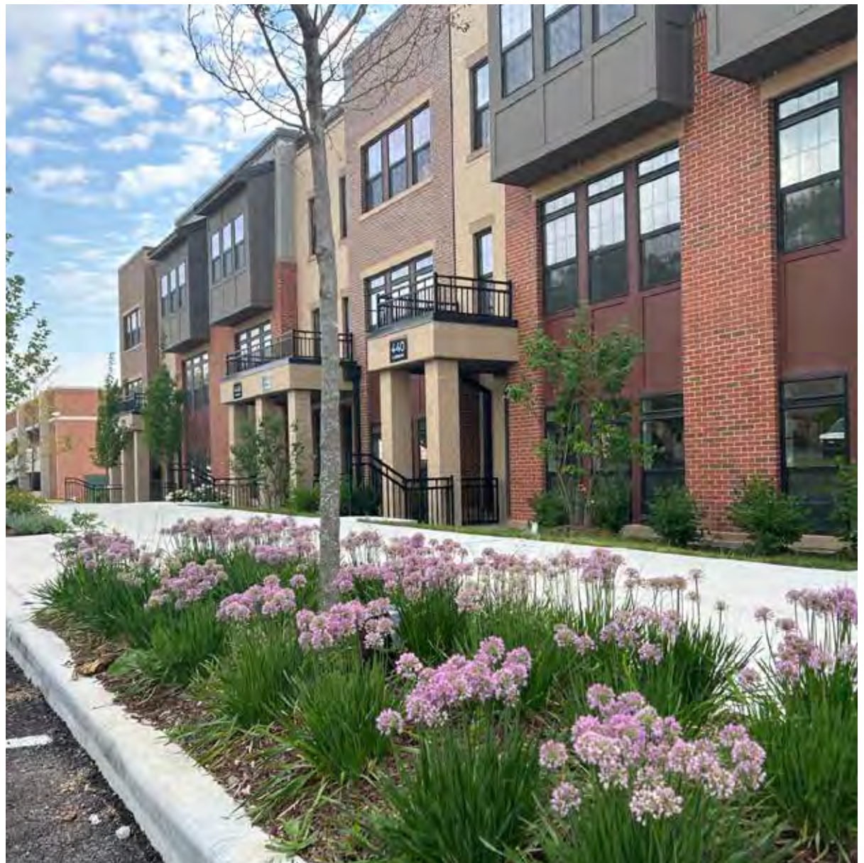
Redevelopment of the former Greenwood Middle School site at 523 S. Madison Avenue into The Madison has significantly boosted assessed value in the downtown.
