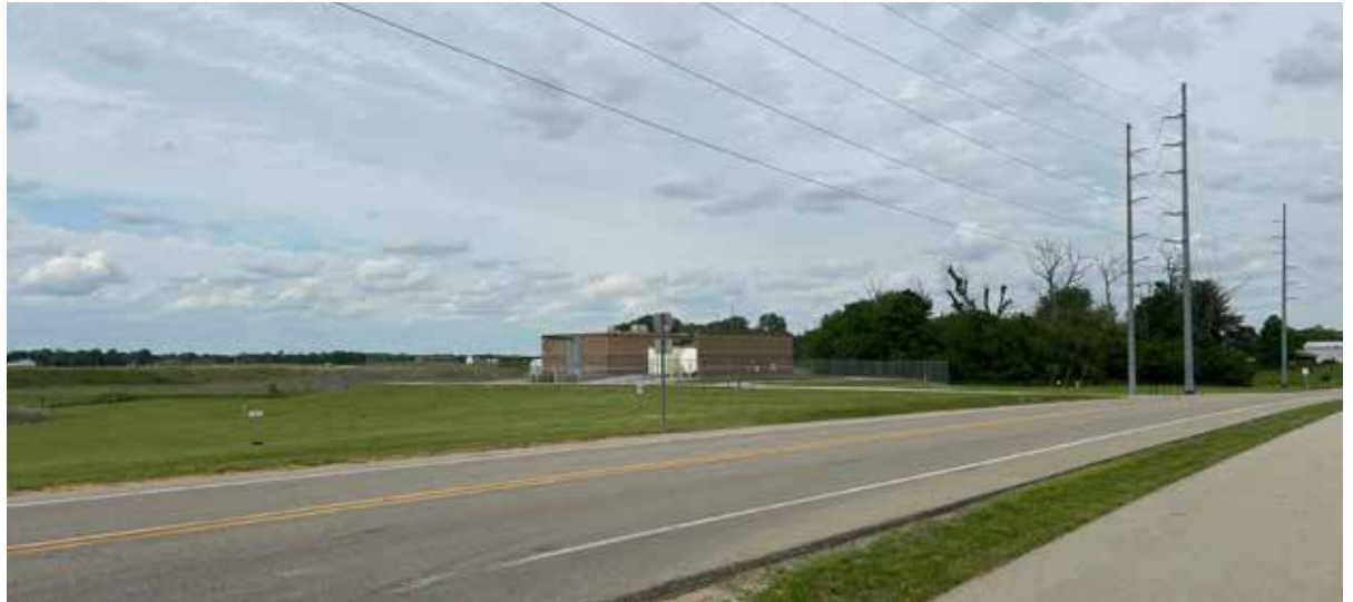
In the response to future growth along the Worthsville Corridor, Greenwood will need to expand utility infrastructure and should actively acquire suitable sites.
