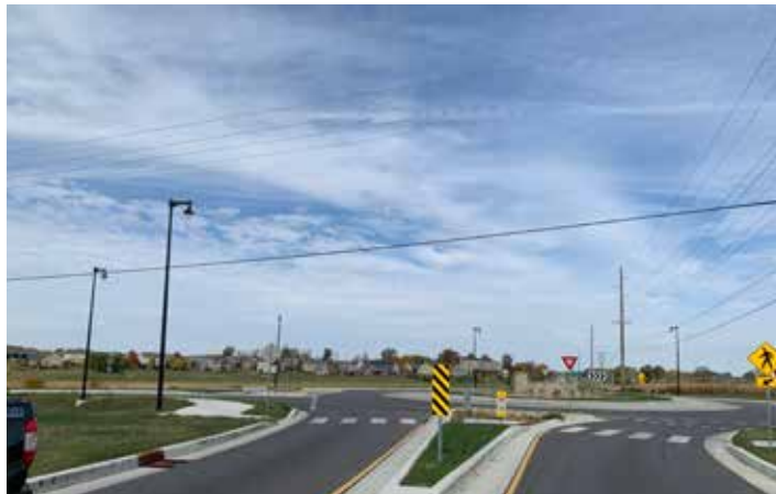
Key roundabouts have helped ease east-west traffic congestion on high-traffic roads.
