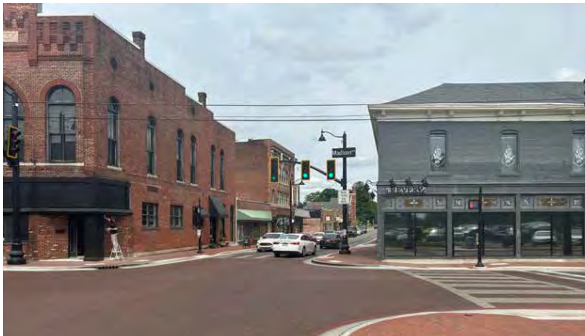
Recent investments in Old Town Greenwood include new brick paver sidewalks, lighting, and furnishings.
