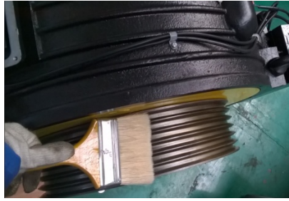
Fig.4 Method of applying anti-rust paint
