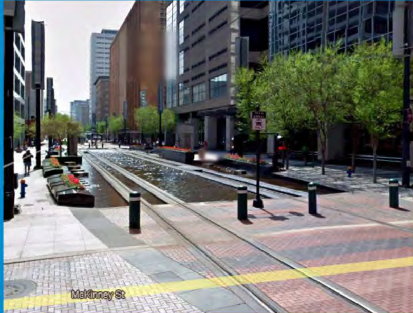
Embedded Track with Pavers
