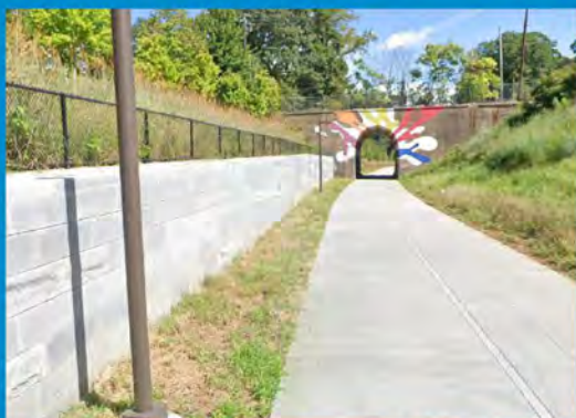
Granite Facing Retaining Wall with Chain-Link Fence
