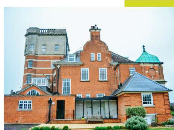
Devitt House building at Pangbourne College
