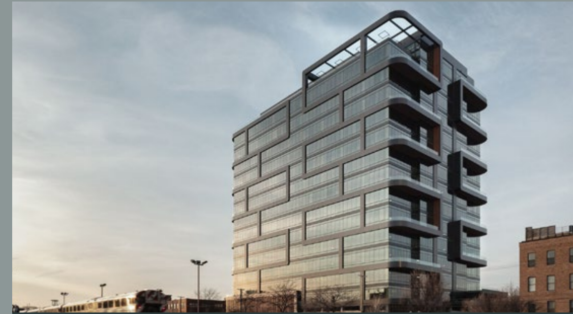
400 N Aberdeen (Delivered 2020)
