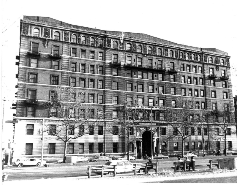
Graham Court Apartments, 1923-1937 Adam Clayton Powell, Jr., Blvd. Clinton & Russell, architects. Built: 1899-1901
