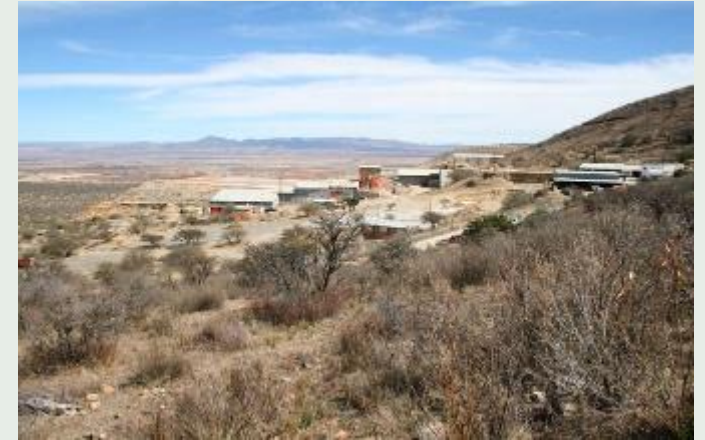
Looking from the west end of the Los Rosarios vein towards the plant, c. 2006
