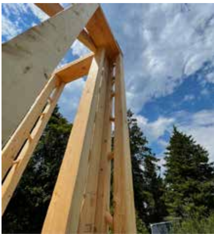
Figure 4. Drywall Nailer in Corner
