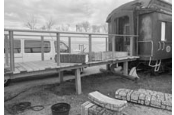
This stage, erected on the grounds of the train station, was erected without a permit and, according to the Township, was not built to code. Photo used with permission from the Township of Uxbridge
