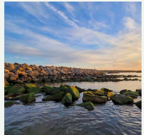
A living breakwater off of Staten Island. Source: SCAPE
