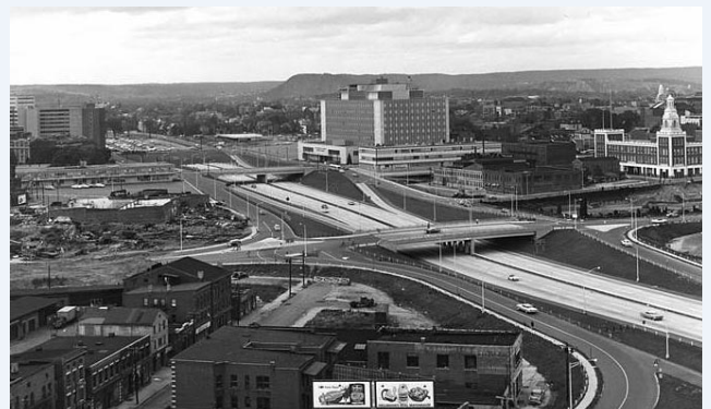
Route 34 shortly after construction
