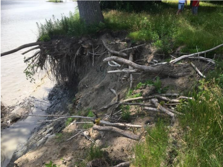
Figure 33. Erosion. Photo taken by author.
