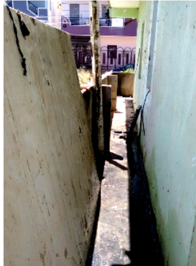
Passage after the intervention
