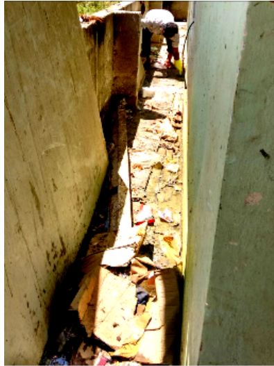
Passage before the intervention
