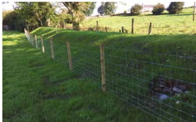
Earth bund to temporarily store runoff during storm events at Greysouthern. A 150 mm pipe through the bund allows the field to drain down after flood events. With thanks to landowner and Greysouthern Parish Council. Image © Cumbria County Council.
