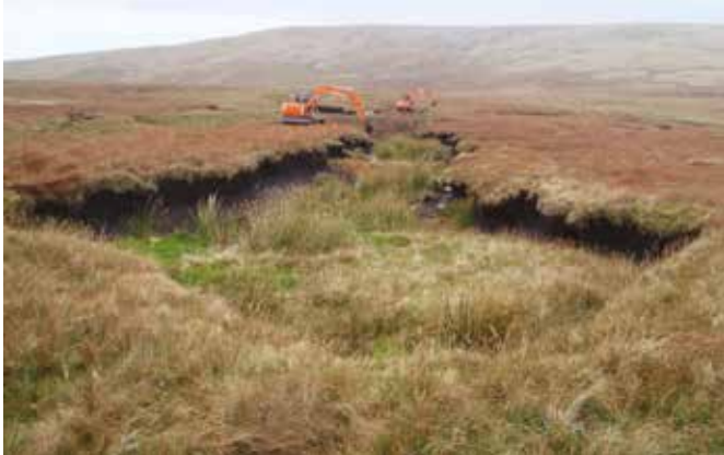
Regrading the steep bank of a peat hag on an area of degraded peat on Kinmont Buckbarrow, near Millom, Cumbria. © Cumbria Wildlife Trust.
