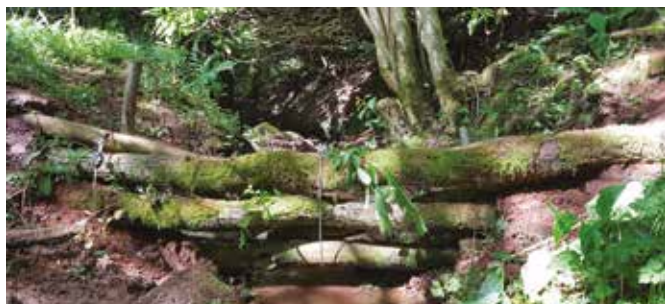
A series of 24 woody dams installed in Cumrew beck to reduce flooding in Cumrew village, near Carlisle. © Eden Rivers Trust
