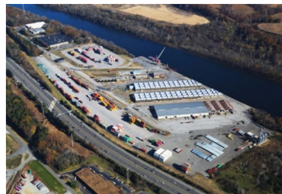
Figure 14. Richmond Marine Terminal
