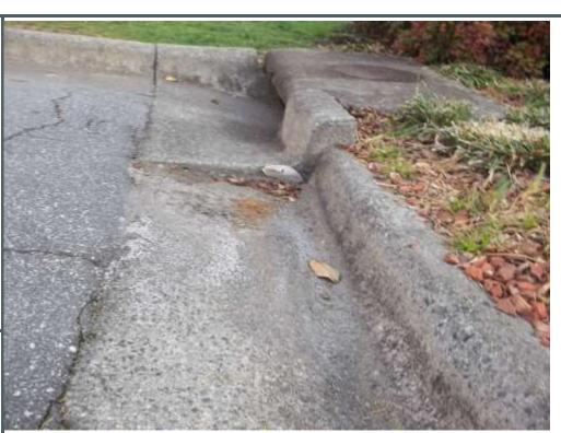
View of spalling/cracking in concrete curbing.
