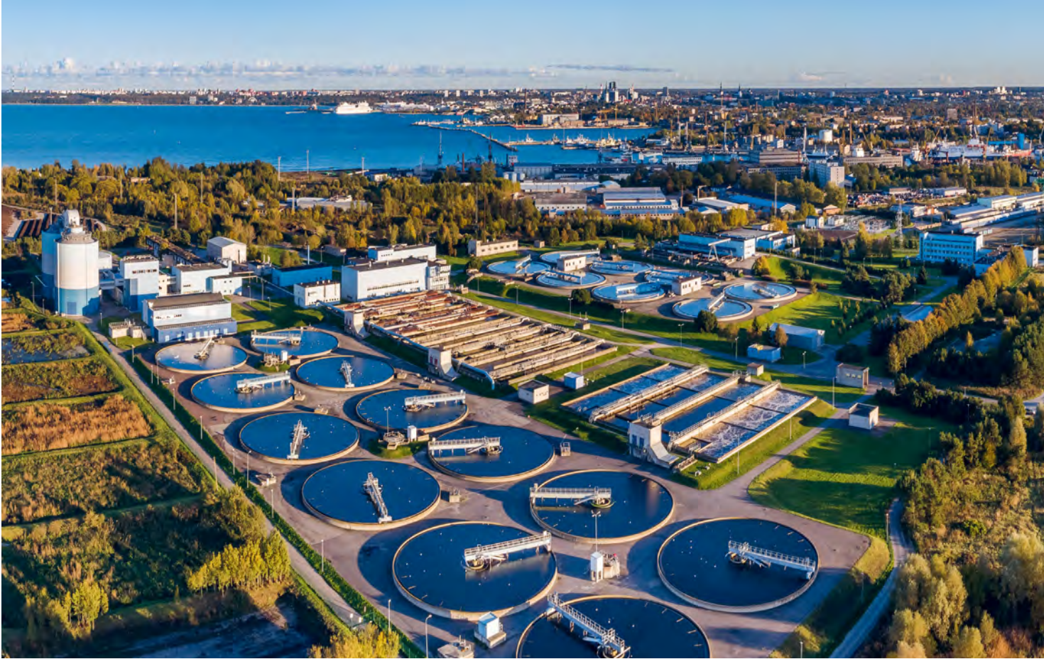
Paljassaare Wastewater Treatment Plant
