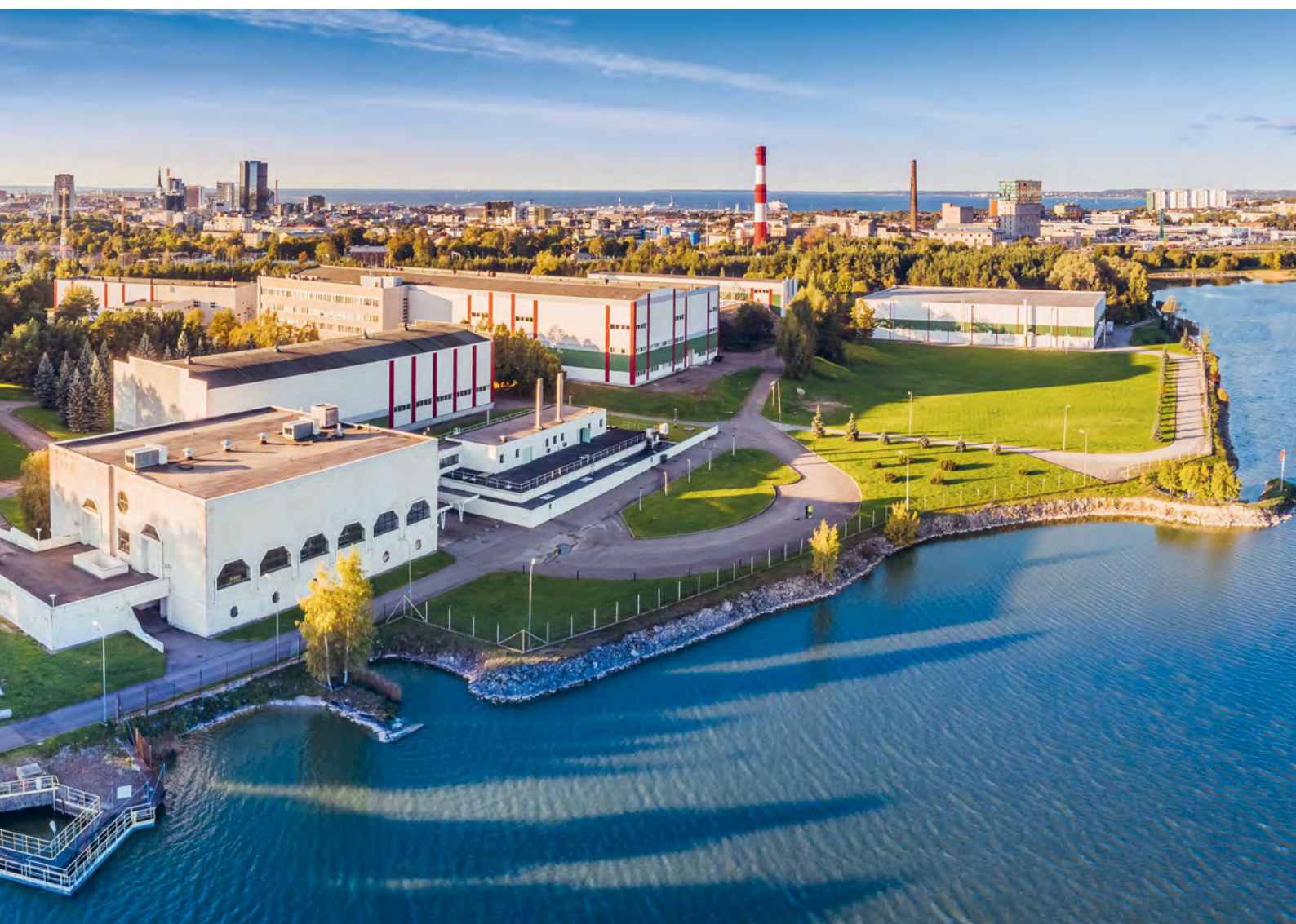
Ülemiste Water Treatment Plant
