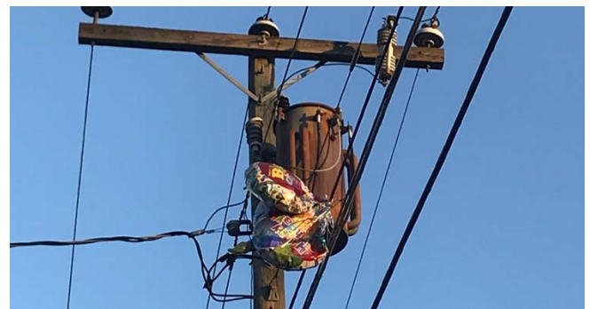
When foil balloons (plastic covered with metallic paint) contact power lines, they cause thousands of customers to lose power. Photo by Katie Register, CVW.
