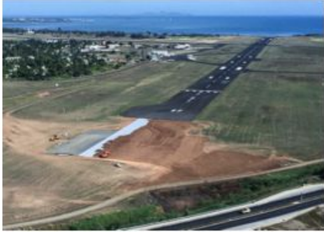
Prepared natural (i.e., soil or grass) compacted open areas
