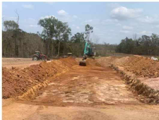
The sediment pond (above) under construction and (right) after 12 months after having filled then evaporated.
