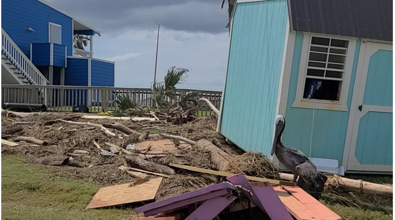
Figure 25: Sargent—Storm Surge Damage
