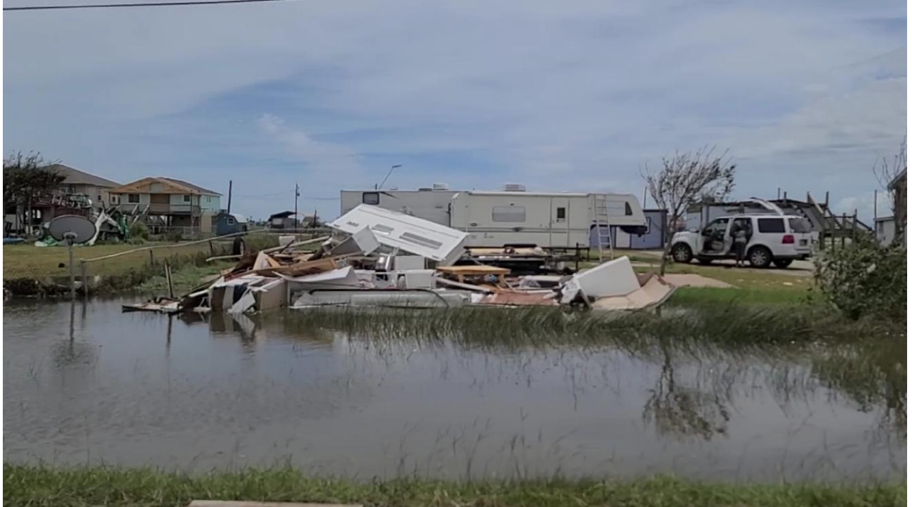
Figure 35: Sargent—Storm Surge Inundation
