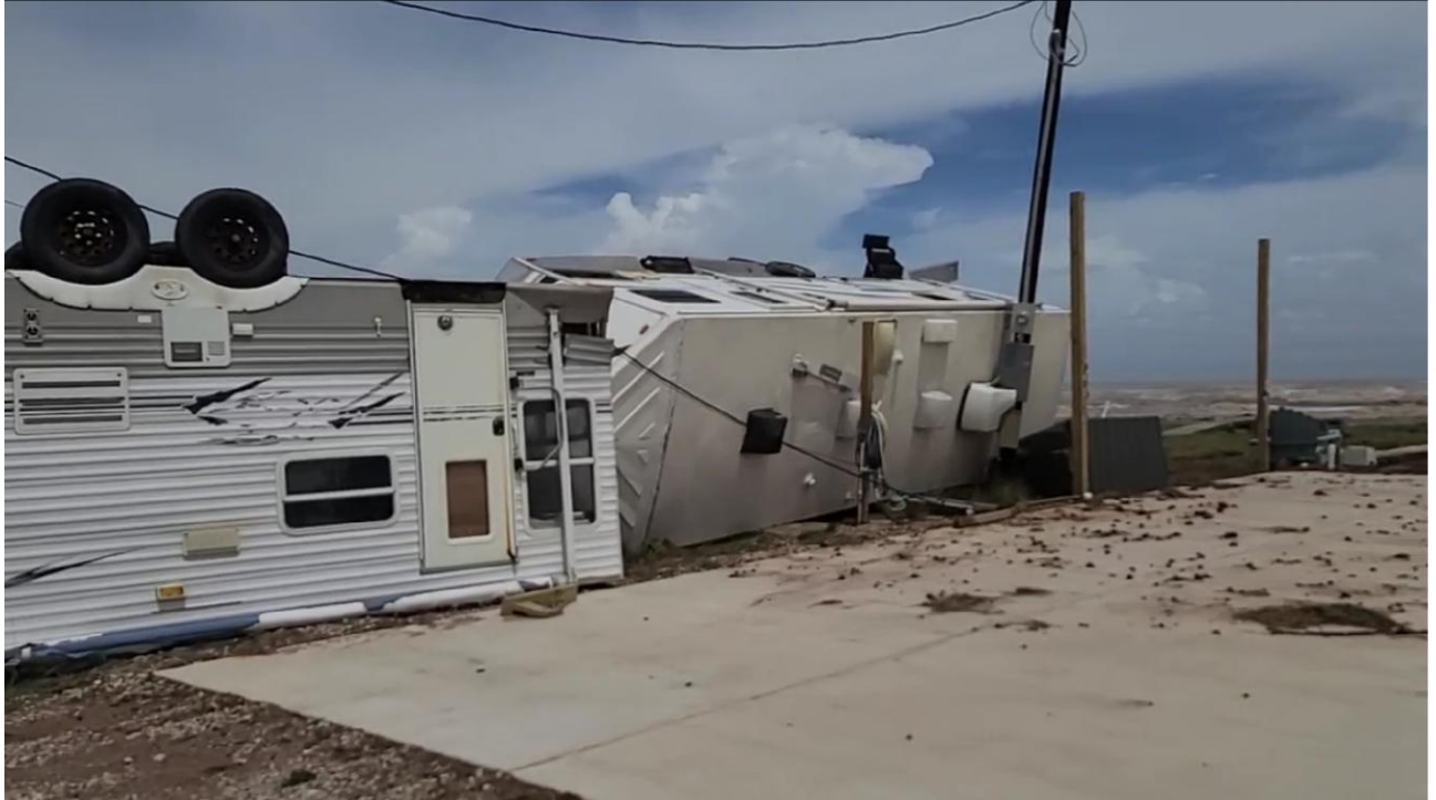
Figure 23: Sargent—Wind & Storm Surge Damage
