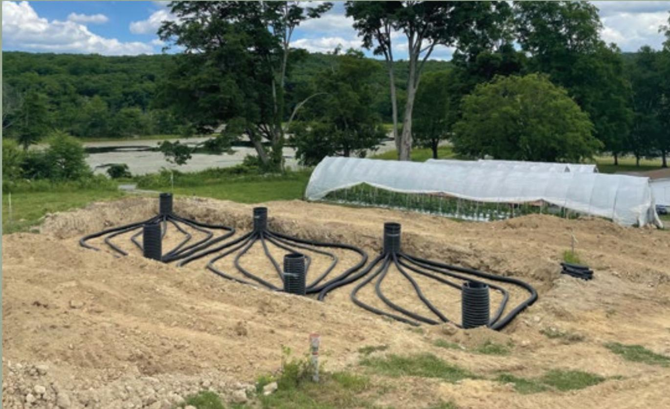
Climate Battery Greenhouse while being constructed—the underground network of pipes distributes the warm air captured above, Credit: Glynwood
