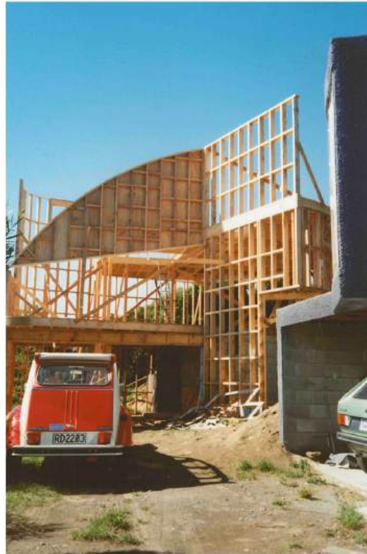
Initial framing installed and start of curved roof side support
