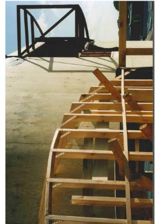
Initial framing installed and start of curved roof side support
