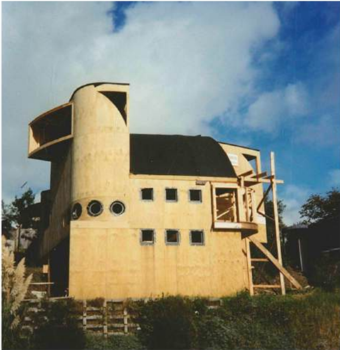
Initial framing installed and start of curved roof side support
